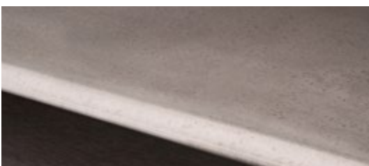
Reinforced concrete plate
